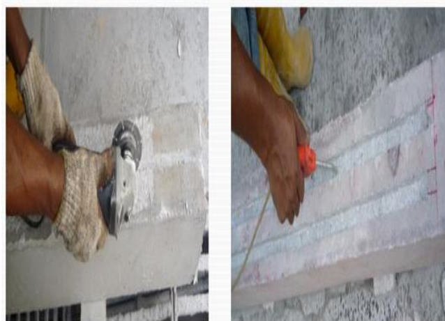
Fig:Cutting and Cleaning of Grooves
