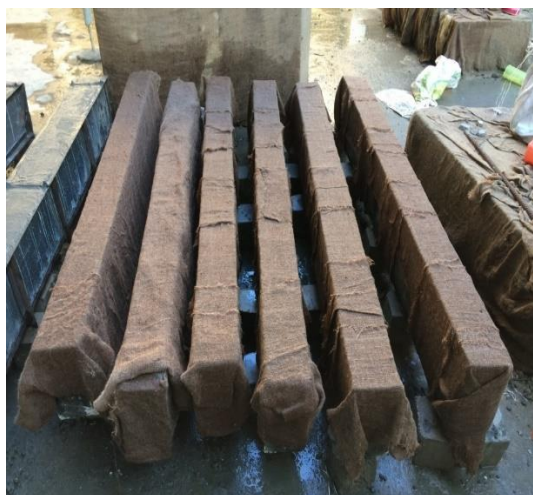
Fig: Curing of Beam
