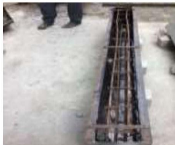
Fig.: Reinforcement Cage
