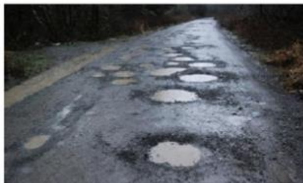
Fig. 1. Potholes on roads [1]
