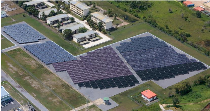
Figure 3: The aerial view of TSB PV power plant
