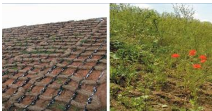
Erosion control by geotextile fiber
