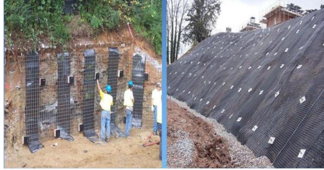
Rock bolting and soil nailing
