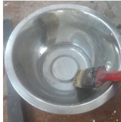
Fig. 4. Mixing of Epoxy and the hardener
